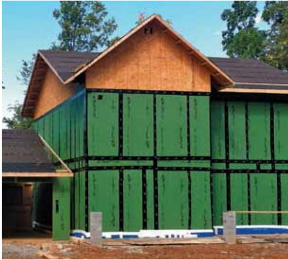
**Exterior insulation eliminates thermal bridging.** The house received a continuous layer of nail-base insulation, which workers fastened to the frame with structural screws and adhesive. Home Slicker Plus Tytar underlayment created a vented rain screen under the fiber-cement siding.
